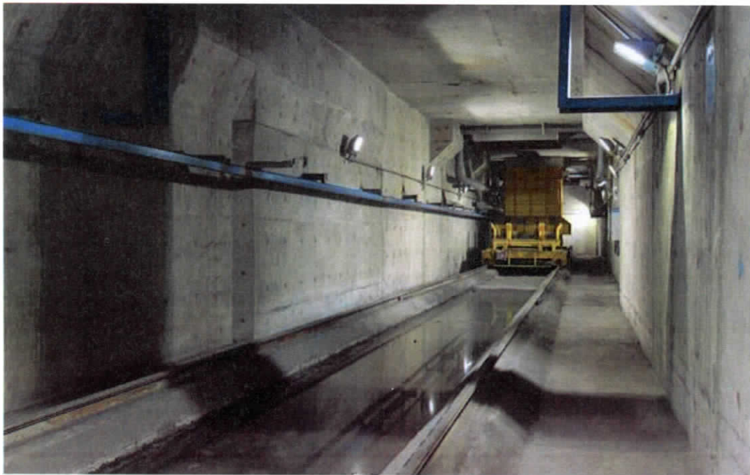
Figure 13. The charging bucket on its way to the lifting point.
