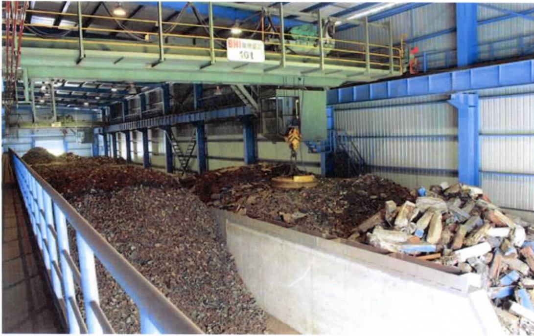
Figure 12: Scrap and skull yard with handling crane
