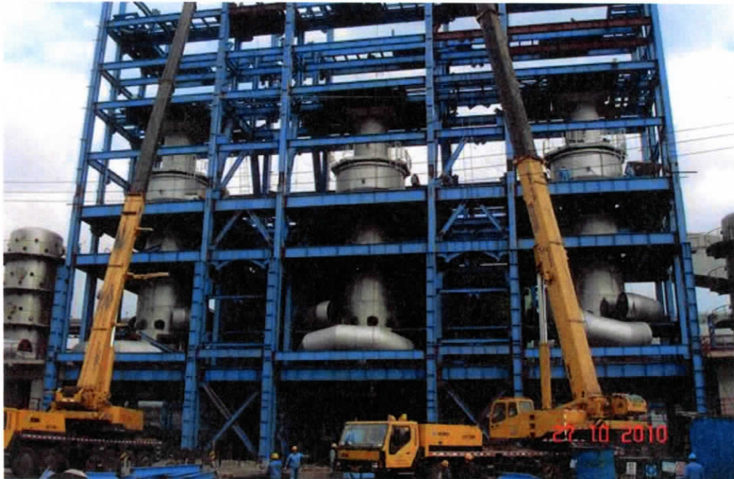
Figure 10. The 3 shaft arrangement during erection
